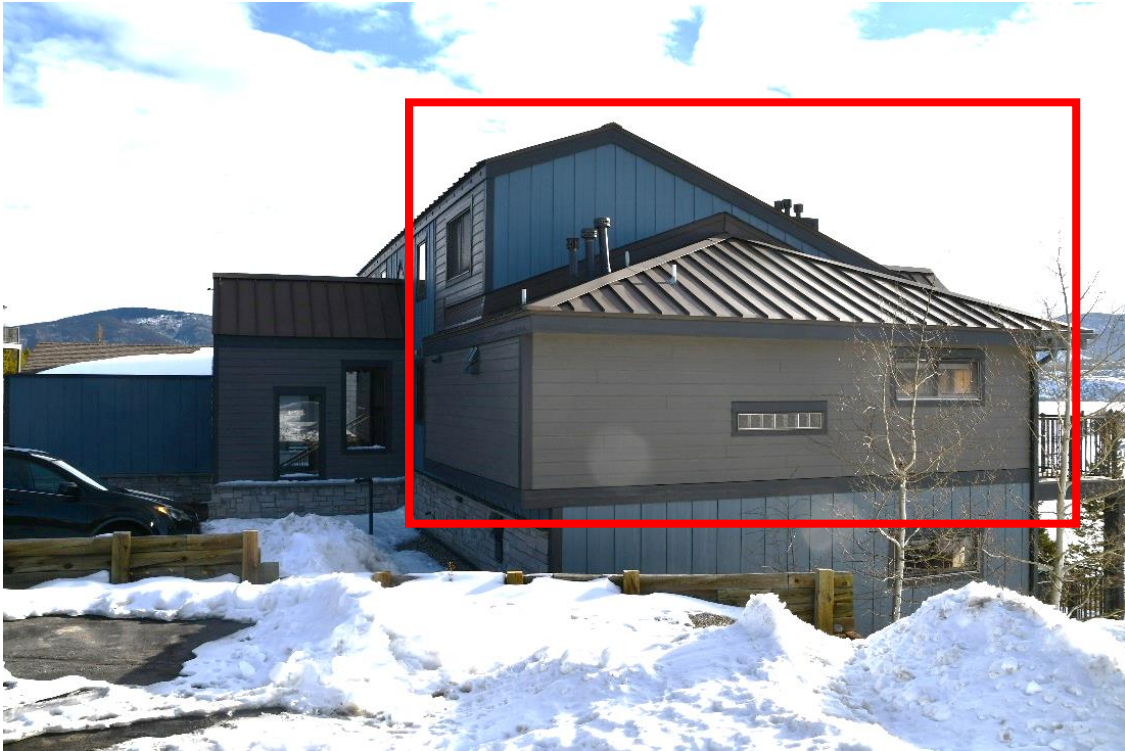
Figure 1. Unit 304B exterior (16020_CBS_1-003).
