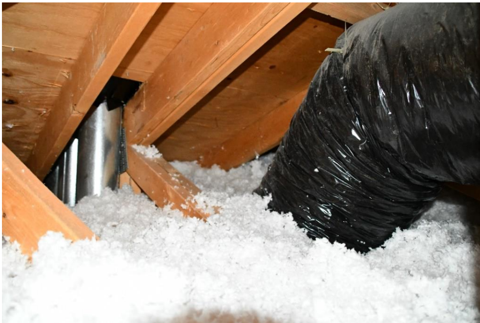
Figure 14. Looking north into the attic from the access panel (16020_CBS_1-078).
