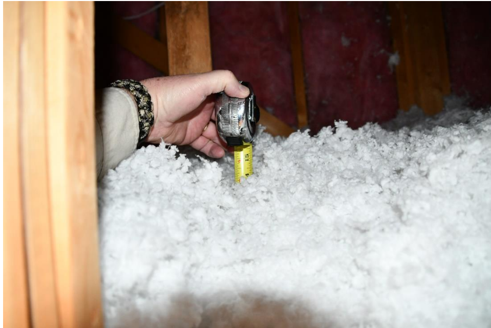
Figure 15. Insulation depth (16020_CBS_1-080).
