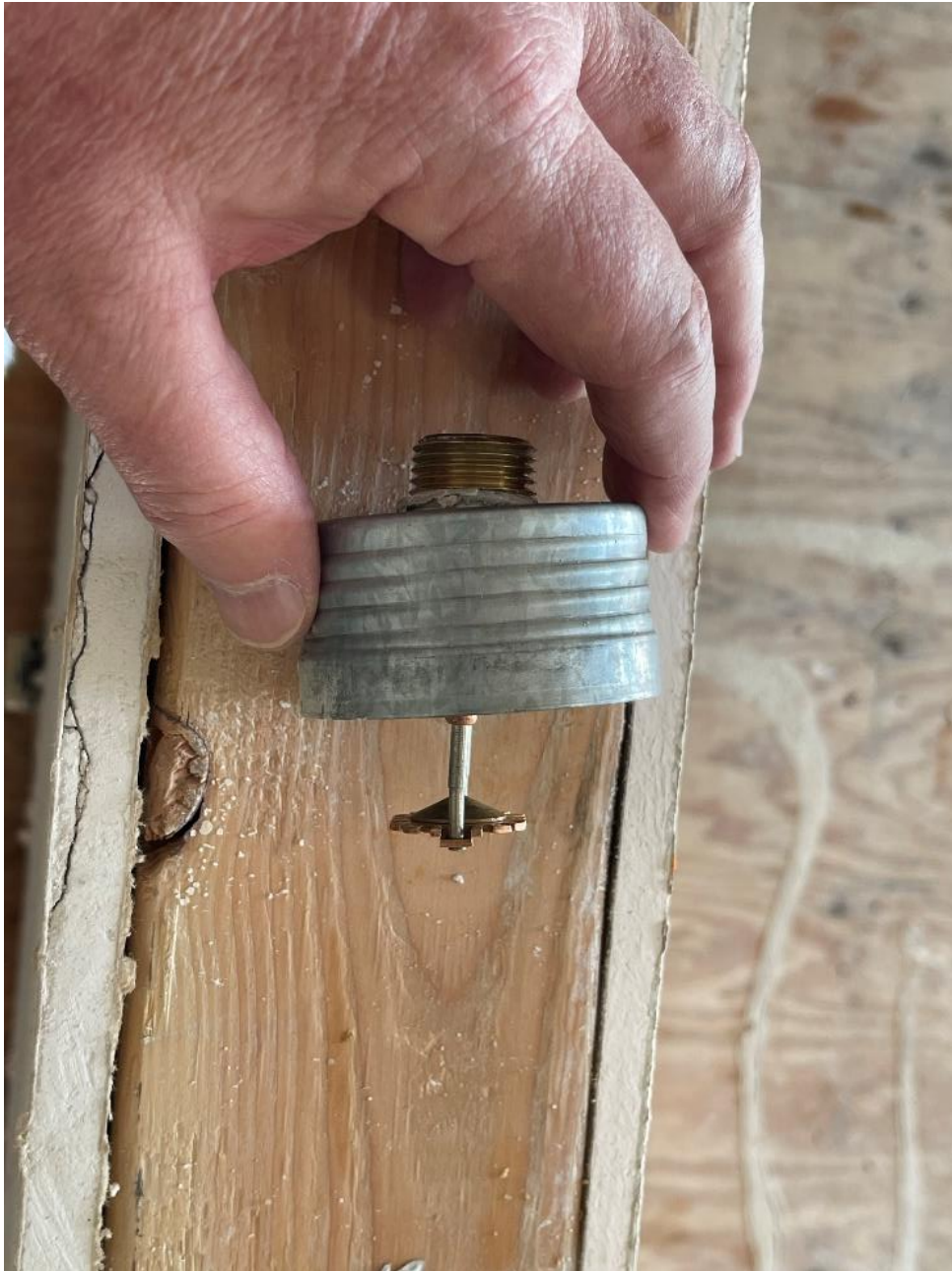
Figure 19. Cup on the subject sprinkler, to which the concealed plate would be assembled (16020_CBS_2-021).
