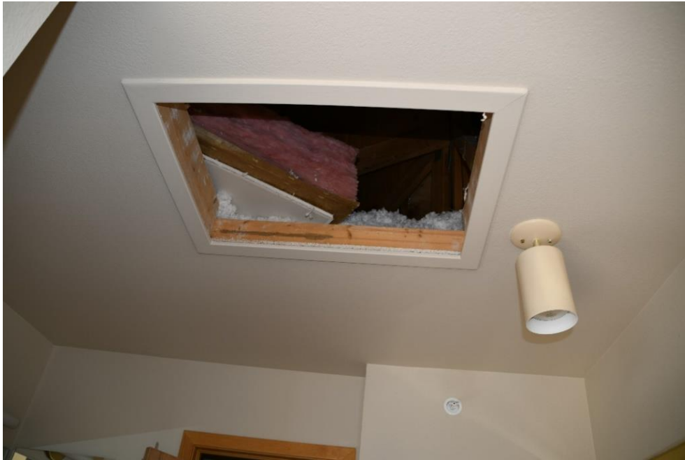
Figure 13. Attic access panel in west bedroom (16020_CBS_1-071).
