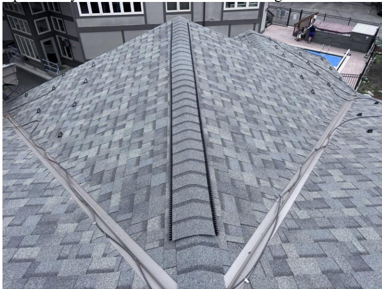
5. W-type open valley metal installed with vented ridge.
