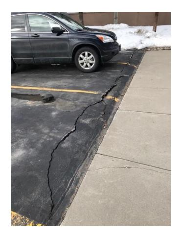
Tim K stated that the concern of the crack that has formed this past winter should be taken care of for preventative maintenance of the parking lot. Noah is going to have this particular area looked at as well have jet black take a look at the rest of the parking lot for cracks that need to be sealed
